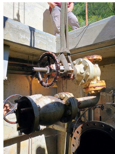
Penstock drain valve assembly removal
