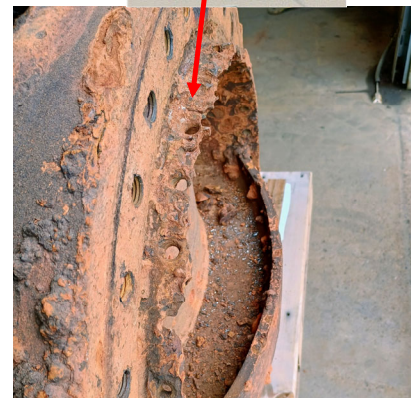
Material will need to be built up in order to redrill and support cap screws for seat alignment
