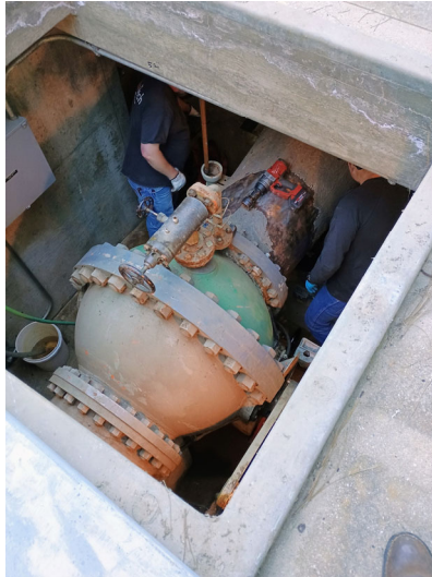
Prep for downstream relief cut
