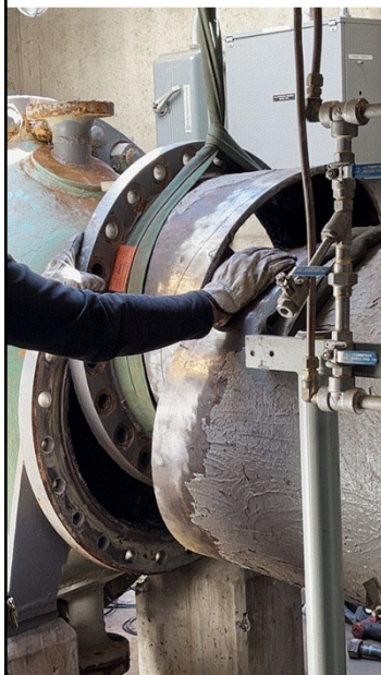
Wedge cut removal
