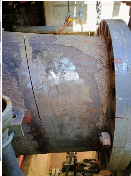
Relief cut needed to allow clearance for valve removal.
