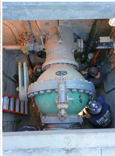
Unbolting from Penstock flange
