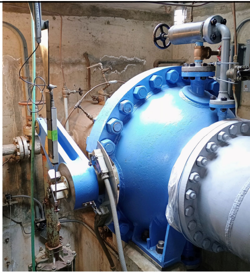
Reinstall the operating arm, the Scroll case charging assembly, and the electrical position devices
