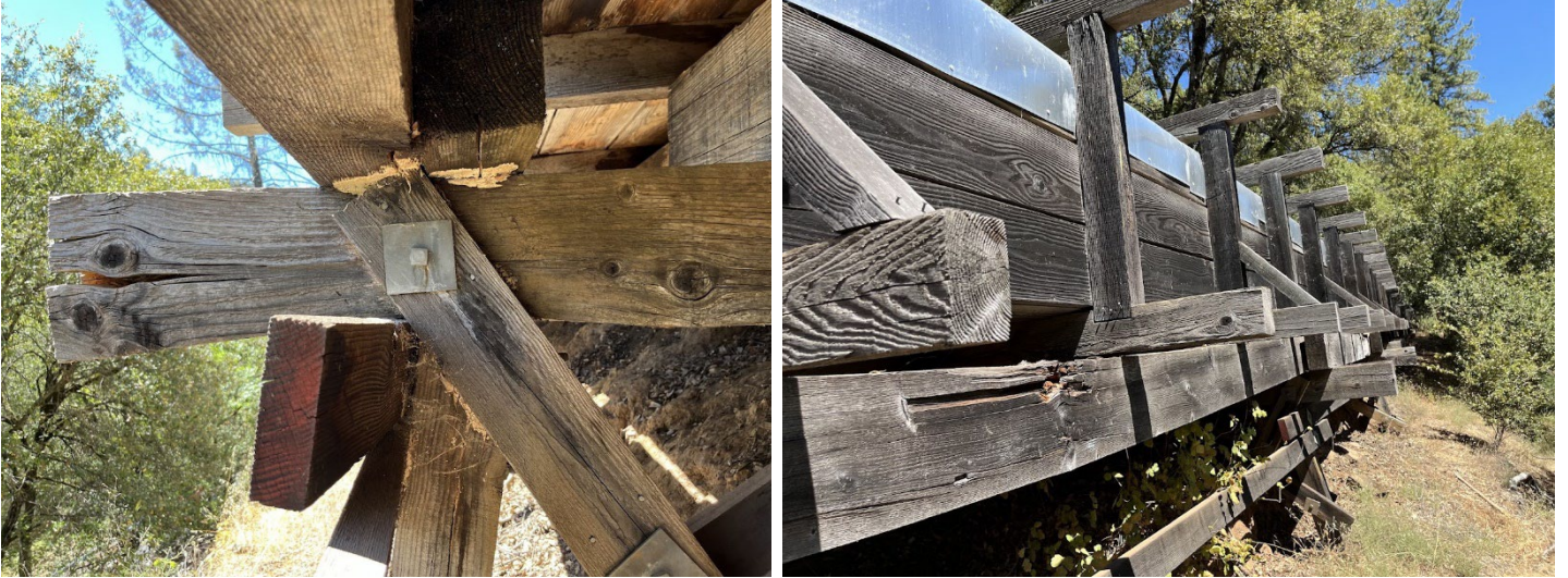
Bent cap replacement on File Flume
