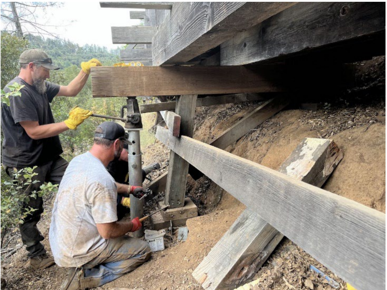
Bent cap replacement on File Flume
