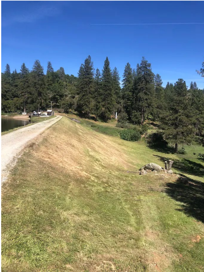
Murphys Forebay South Dam
