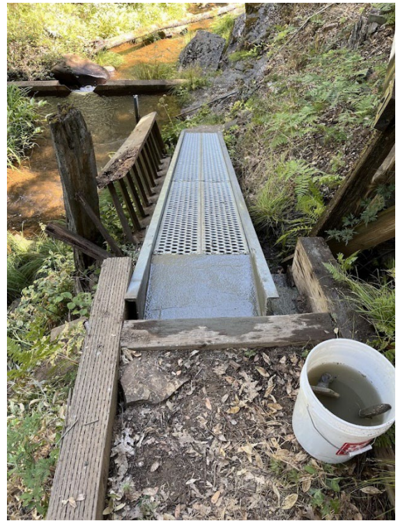
Metal walk ramp down to S128
