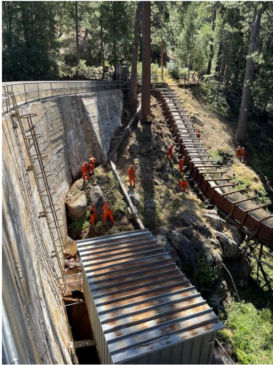
Vegetation control at Hunter Dam
