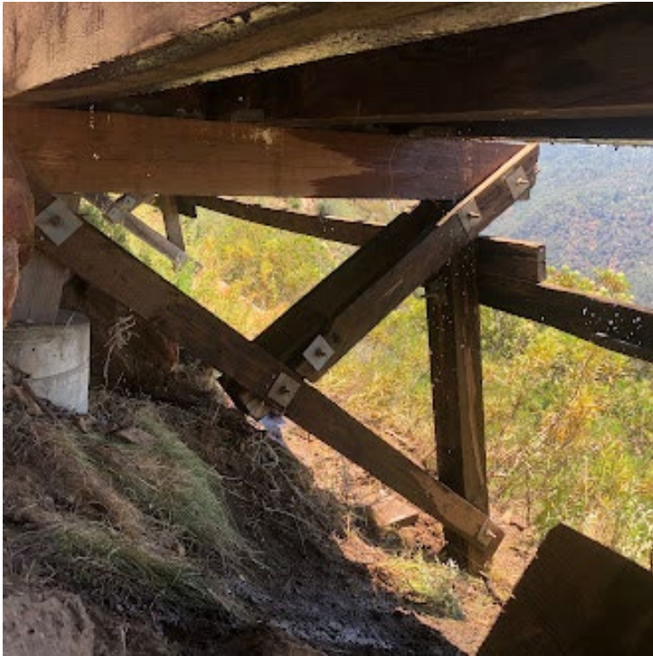
Bent replacement at \frac{3}{4} mile flume
