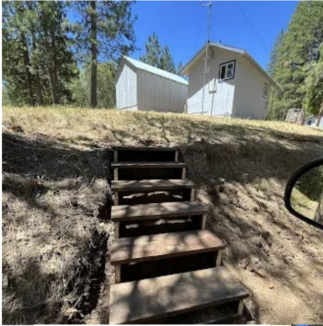
Stairs to saw shop at Hunters
